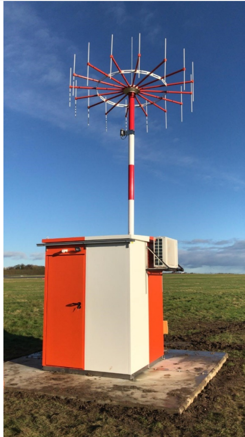
Figure 4 - VDF Shelter Installation at Cambridge Airport, UK.
